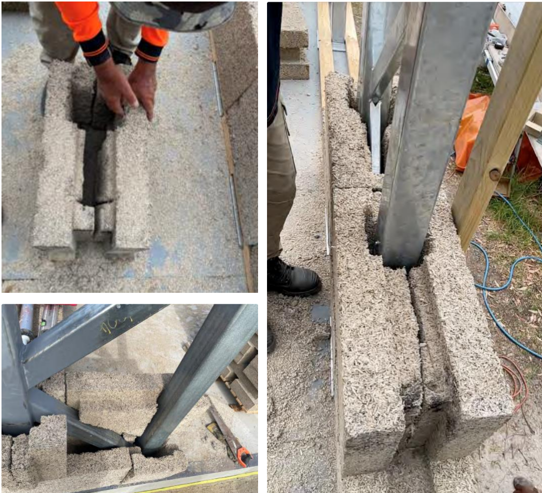
Figure 51 - Encasing a K-brace
