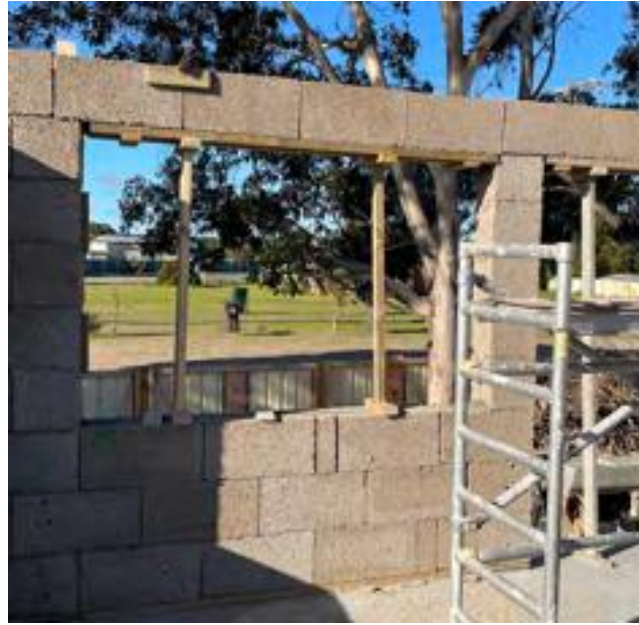
Figure 71 - Placing U-blocks
