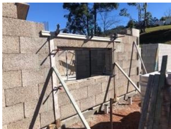
Figure 72 - Safety struts on incomplete walls
