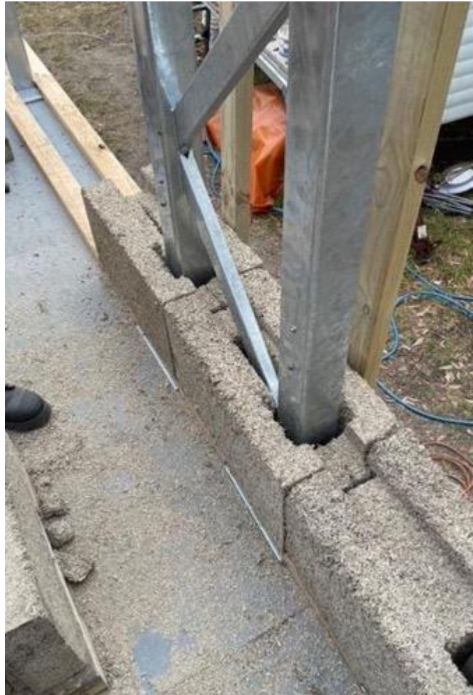
Figure 28 - K-brace installation
