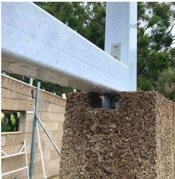
Figure 64 - FRP window lintel supporting blocks
