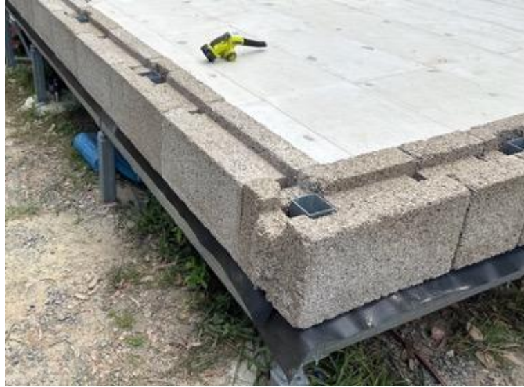
Figure 19 - Fire resistant magnesium board floor
