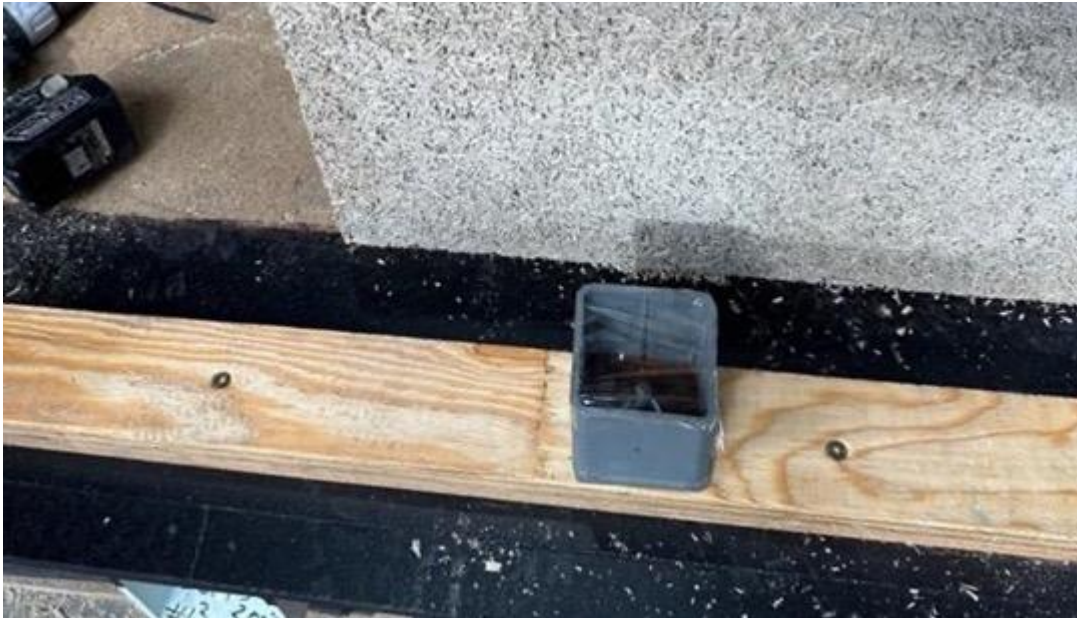
Figure 20 - Tongue, stanchion on timber floor
