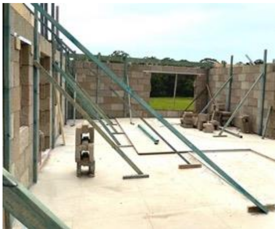
Figure 72 - Safety struts on incomplete walls
