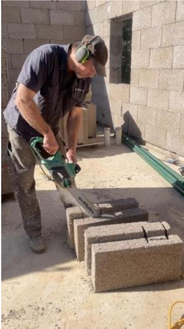
Figure 33 - Cutting a column hole
