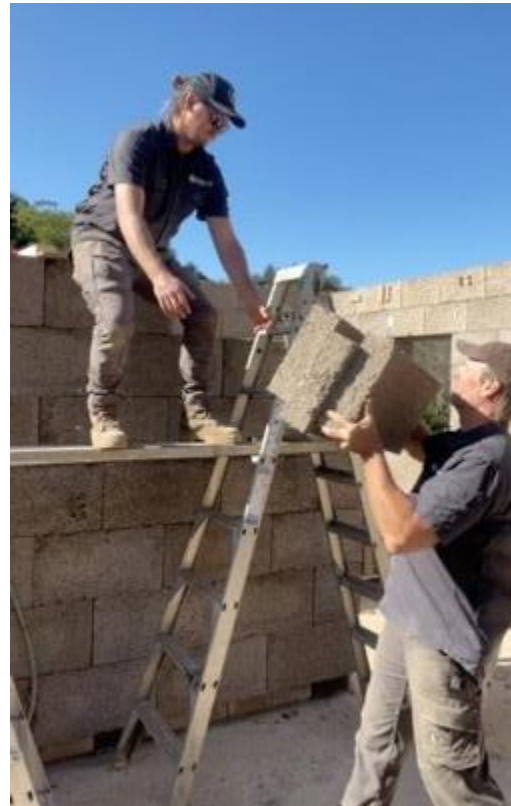
Figure 31 - How to pass a HempBLOCK
