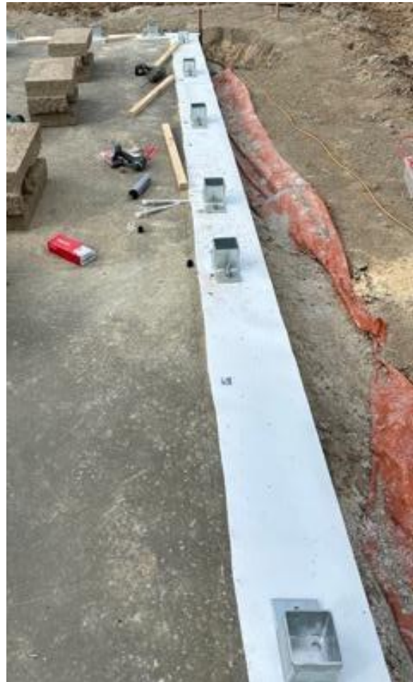
Figure 25 - Waterproofing and termite proofing in one
