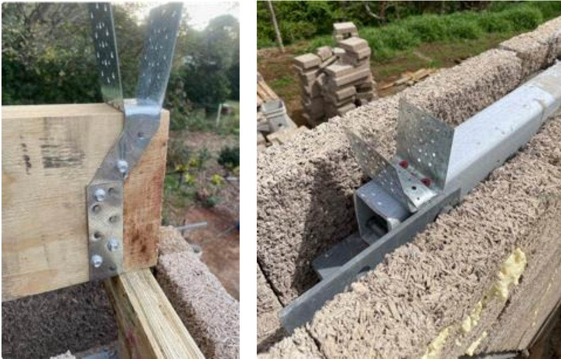
Figure 75 - Burman roof anchor brackets
