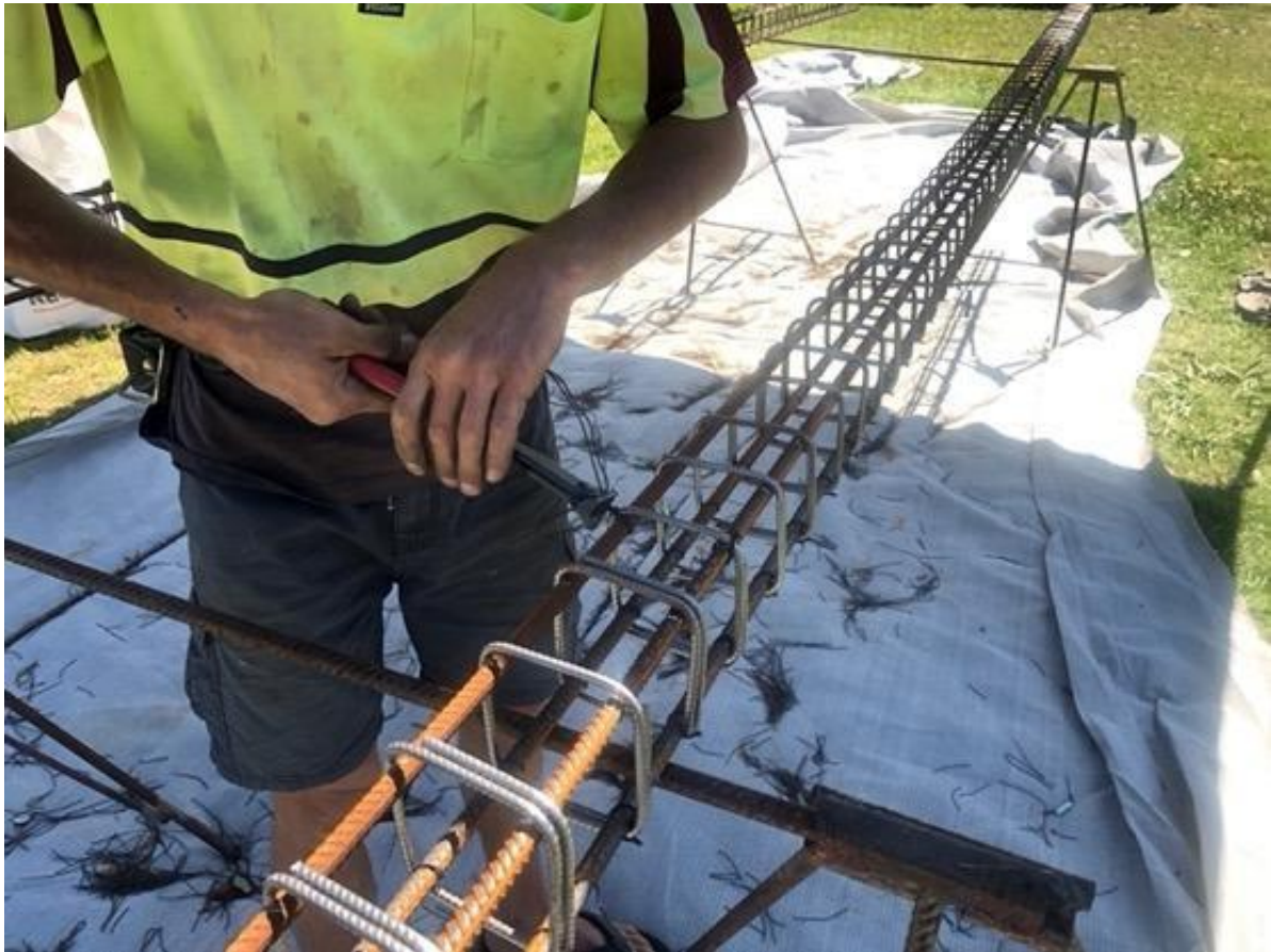
Figure 77 - Making steel cages
