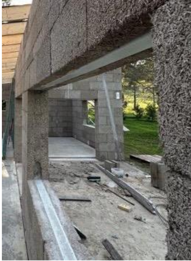
Figure 65 - Lintel (header) supporting blocks
