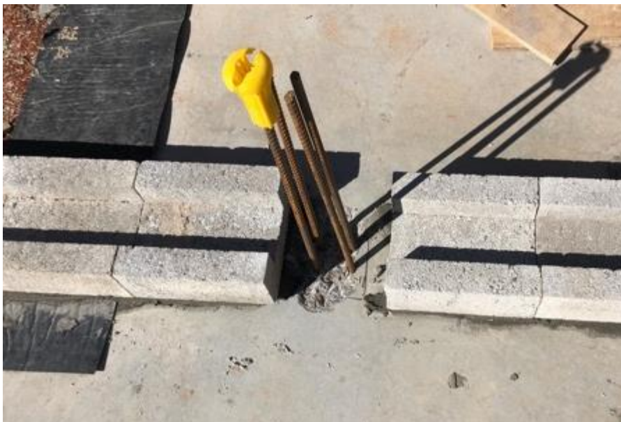
Figure 30 - Concrete starter blocks
