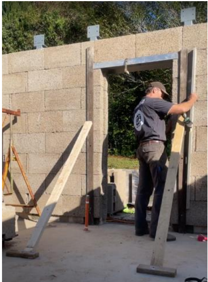
Figure 66 - Bracing and checking a wall for plumb before casting perlite
