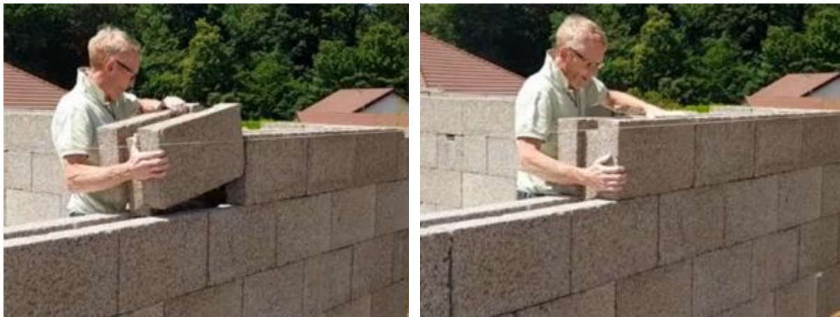
Figure 48 - Stacking blocks
