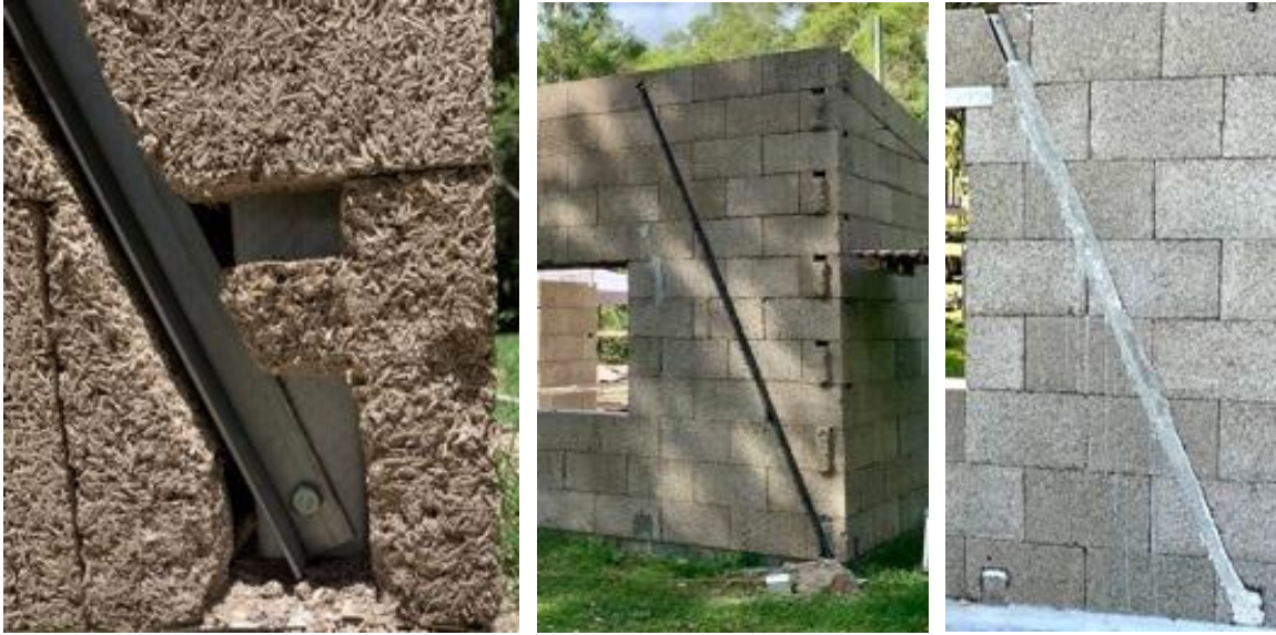
Figure 59 - A diagonal braces
