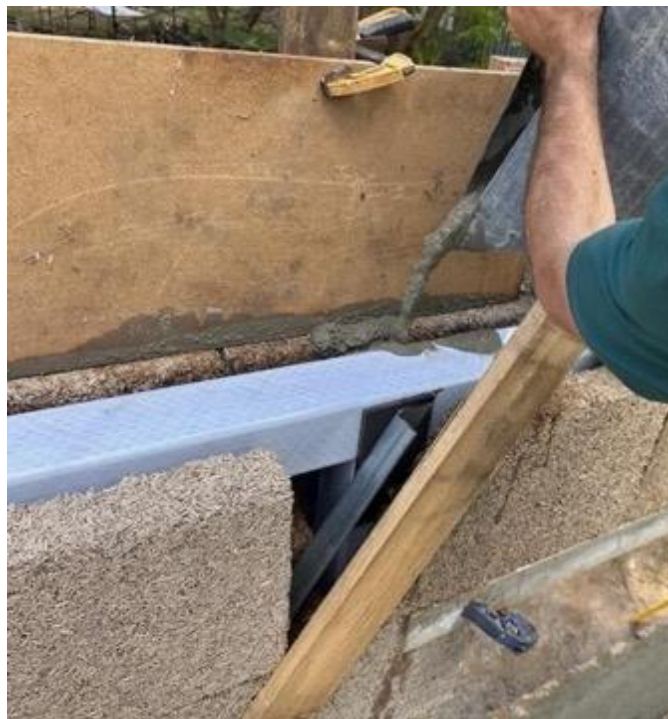
Figure 76 - Mixing and placing a perlite-cement mix
