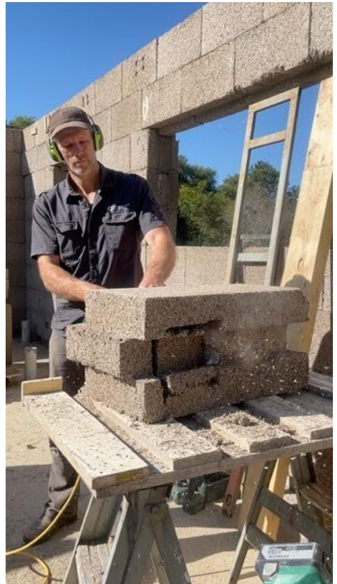
Figure 33 - Cutting a column hole
