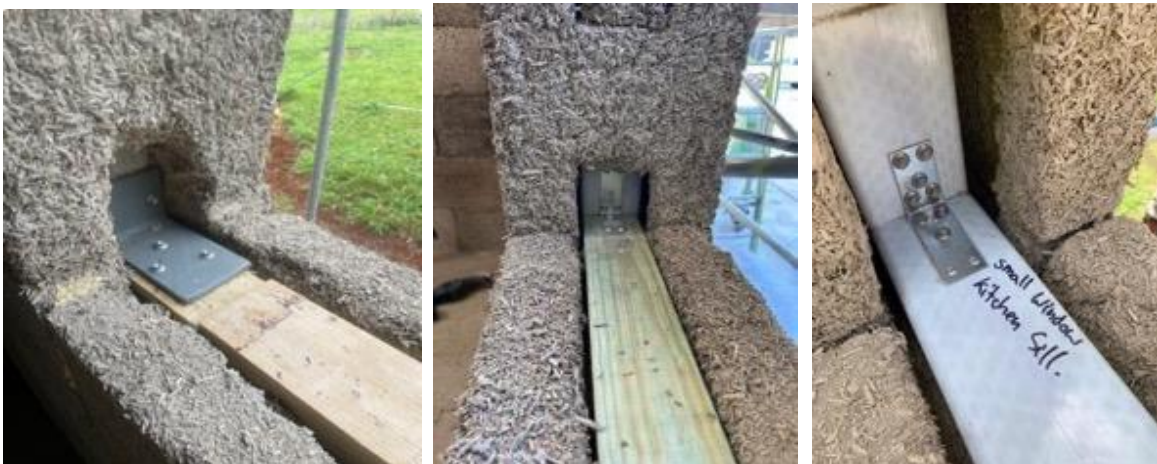
Figure 60 - Installing windowsills
