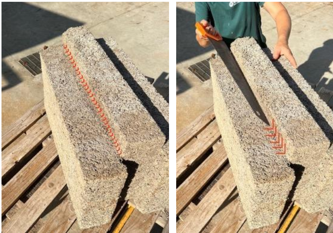
Figure 6 - Shaving the edge of the tongue
